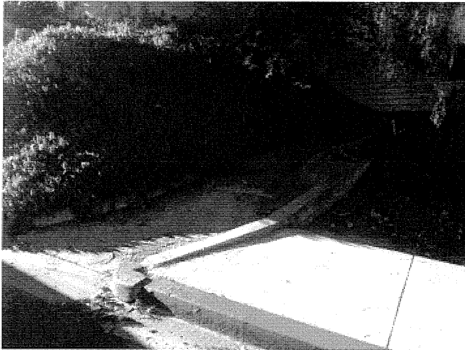
Concrete Spillway on S. Nardo Avenue
