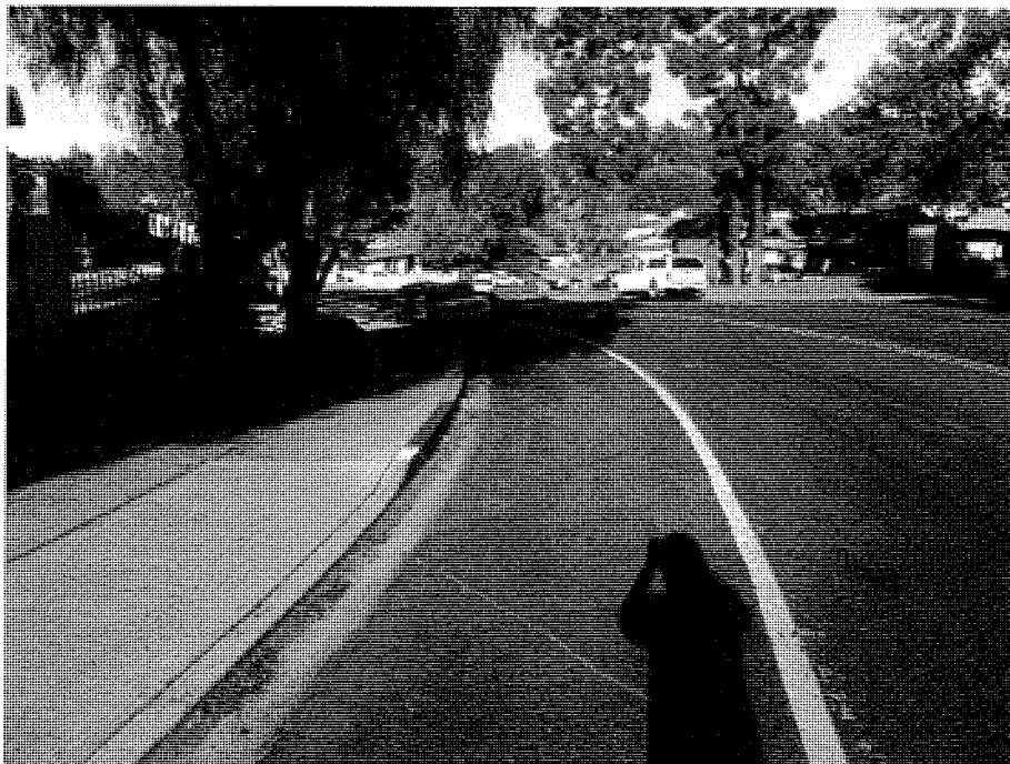
View Looking East along S. Nardo Avenue
